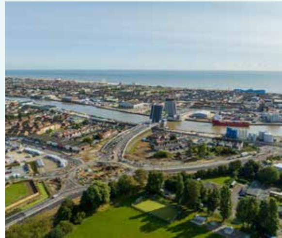
Herring Bridge, Great Yarmouth
