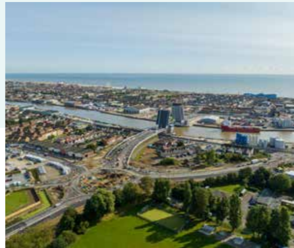
Herring Bridge, Great Yarmouth
